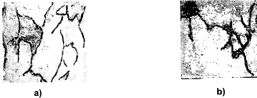
Figure 6.14 Concrete blocks cured with woven of 370 and 700 GSM fabric. a) Woven fabric of 370 gsm, b) Woven fabric of 700 gsm.
