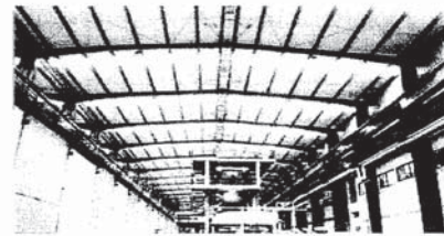
Fig 7.7 Translucent Sheets Inside Sheds
